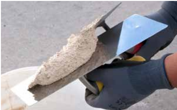
3. Colocar PX-28 Isolxtrem SILOXANE TECHNOLOGY M na talocha.
