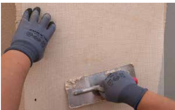
7. Colocar a malha RG-116 Isolxtrem System.
