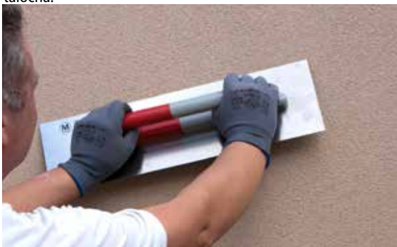
5. Alisar o PX-28 Isolxtrem SILOXANE TECHNOLOGY M.
