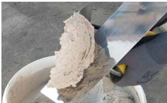
3. Colocar o PX-28 Isolxtrem SILOXANE TECHNOLOGY L na talocha.
