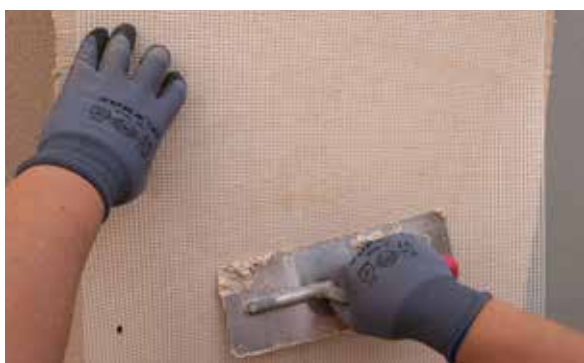
7. Colocar a malha RG-116 Isolxtrem System.
