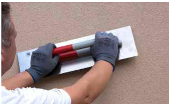
5. Alisar o PX-28 Isolxtrem SILOXANE TECHNOLOGY L.
