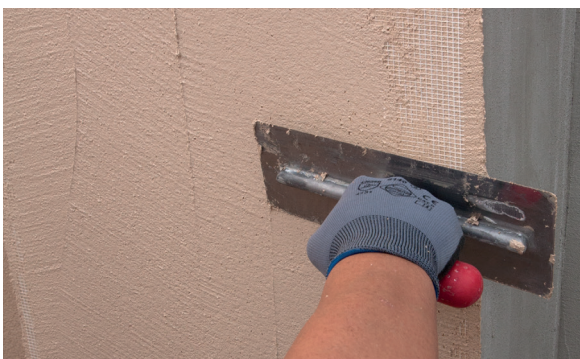
9. Smooth the PX-28 Isolxtrem SILOXANE TECHNOLOGY L deposited on the mesh.
