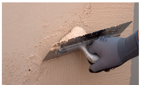
4. Apply PX-28 Isolxtrem SILOXANE TECHNOLOGY L on the surface.
