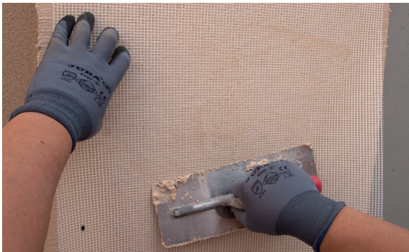
7. Lay the RG-116 Isolxtrem System mesh.
