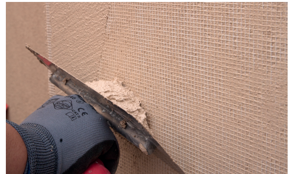
8. Cover the screen with PX-28 Isolxtrem SILOXANE TECHNOLOGY L
