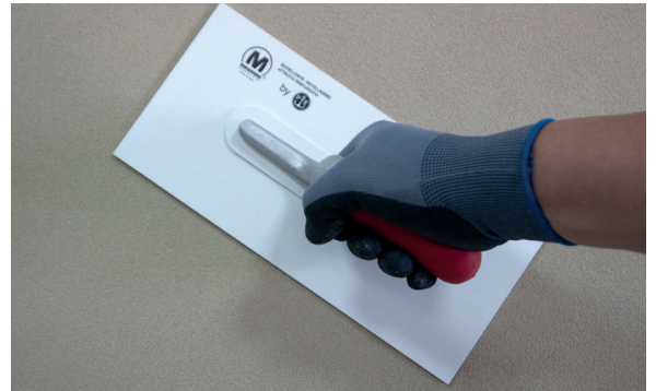
6. Trowel the PX-28 Isolxtrem SILOXANE TECHNOLOGY L
