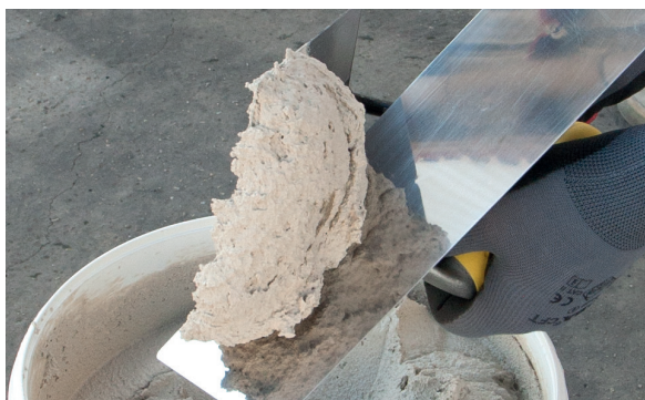
3. Place PX-28 Isolxtrem SILOXANE TECHNOLOGY L on the trowel.
