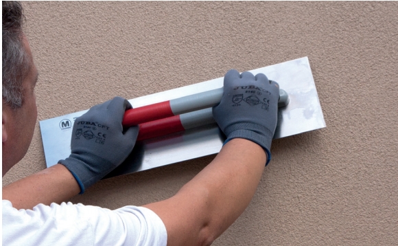
5. Smooth the PX-28 Isolxtrem SILOXANE TECHNOLOGY L
