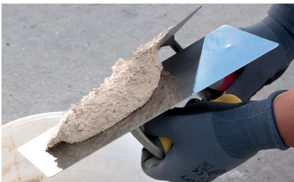
3. Place PX-28 Isolxtrem SILOXANE TECHNOLOGY G on the trowel.
