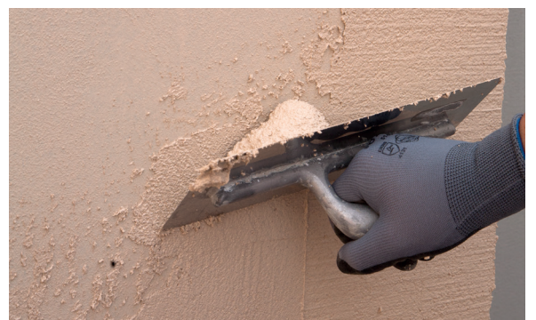
4. Apply PX-28 Isolxtrem SILOXANE TECHNOLOGY G on the surface.
