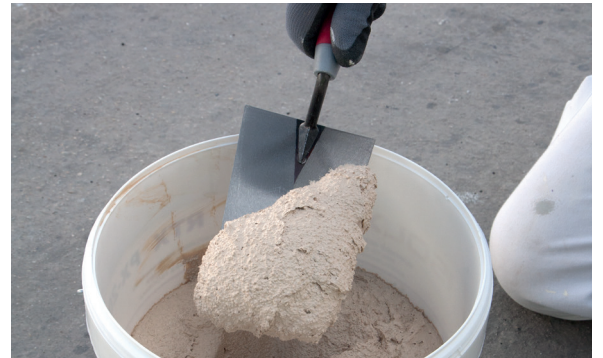
2. Remove the PX-28 Isolxtrem SILOXANE TECHNOLOGY G with the help of a pallet.
