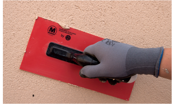
6. Trowel the PX-28 Isolxtrem SILOXANE TECHNOLOGY G
