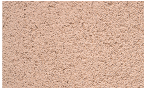
10. Final finishing of the PX-28 Isolxtrem SILOXANE TECHNOLOGY G
