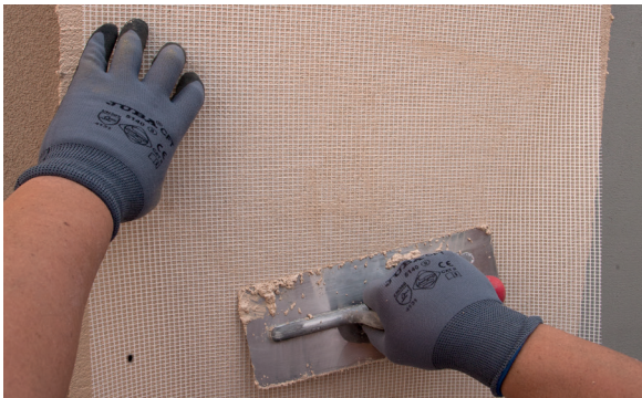
7. Lay the RG-116 Isolxtrem System mesh.
