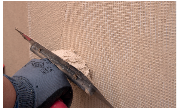
8. Cover the screen with PX-28 Isolxtrem SILOXANE TECHNOLOGY G
