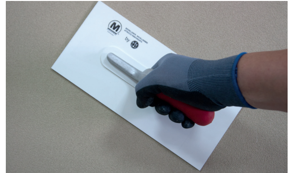
6. Trowel the PX-28 Isolxtrem SILOXANE TECHNOLOGY F.
