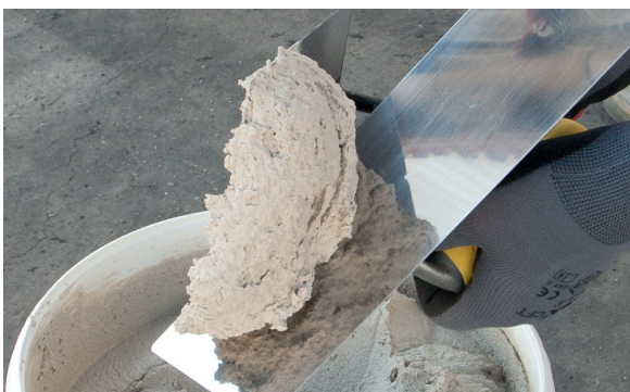
3. Place PX-28 Isolxtrem SILOXANE TECHNOLOGY F. on the trowel.
