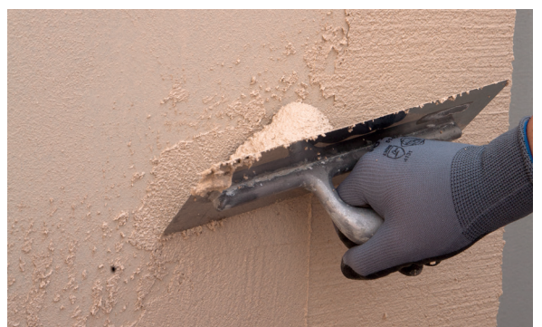
4. Apply PX-28 Isolxtrem SILOXANE TECHNOLOGY F. on the surface.
