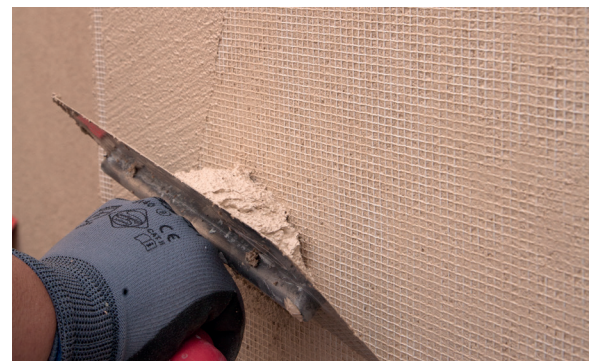
8. Cover the screen with PX-28 Isolxtrem SILOXANE TECHNOLOGY F.
