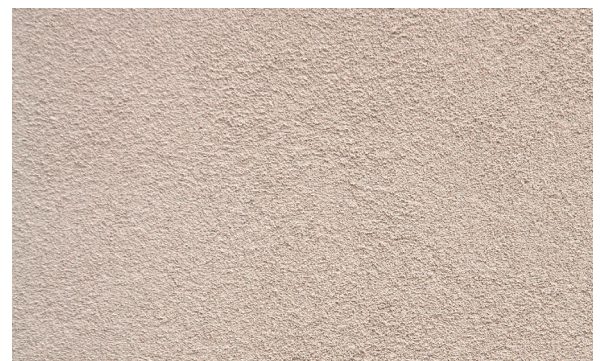
10. Final finishing of the PX-28 Isolxtrem SILOXANE TECHNOLOGY F.
