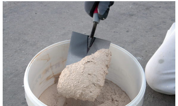
2. Remove the PX-20 Isolxtrem RTX M with the help of a pallet.
