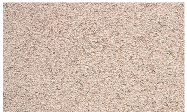
10. Final finishing of the PX-20 Isolxtrem RTX M.
