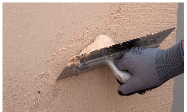
4. Apply PX-20 Isolxtrem RTX M on the surface.
