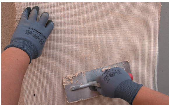
7. Colocar la malla RG-116 Isolxtrem System.
