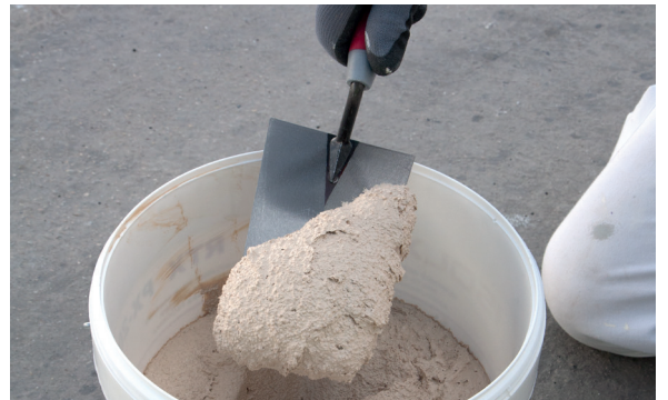
2. Remove the PX-20 Isolxtrem RTX G with the help of a pallet.
