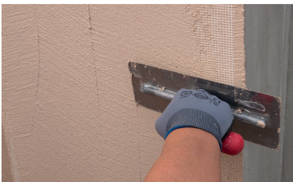
9. Smooth the PX-20 Isolxtrem RTX G deposited on the mesh.
