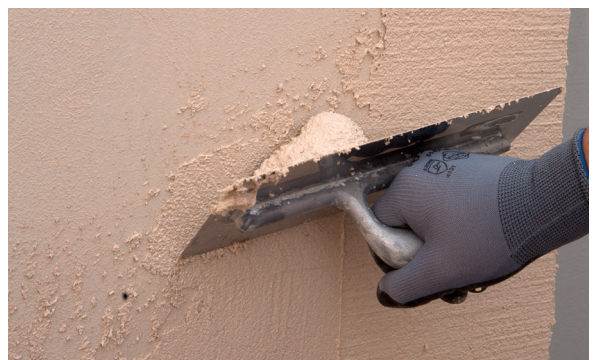
4. Apply PX-20 Isolxtrem RTX G on the surface.
