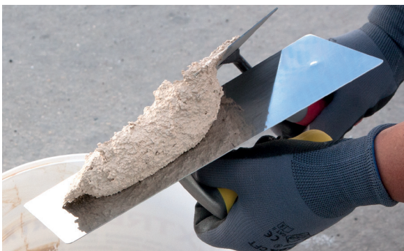
3. Place PX-20 Isolxtrem RTX F on the trowel.
