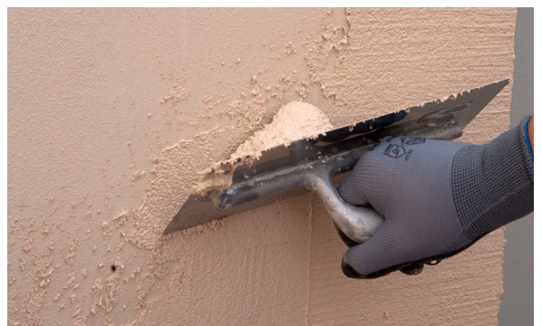
4. Apply PX-20 Isolxtrem RTX F on the surface.
