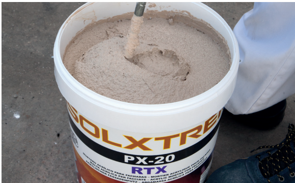
1. Remove the PX-20 Isolxtrem RTX F before use.
