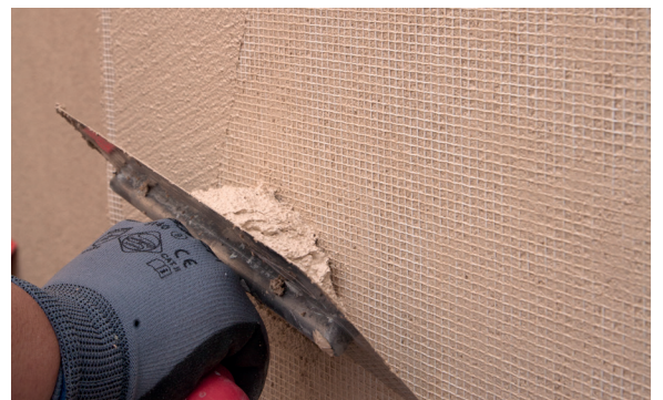
8. Cover the screen with PX-20 Isolxtrem RTX F.
