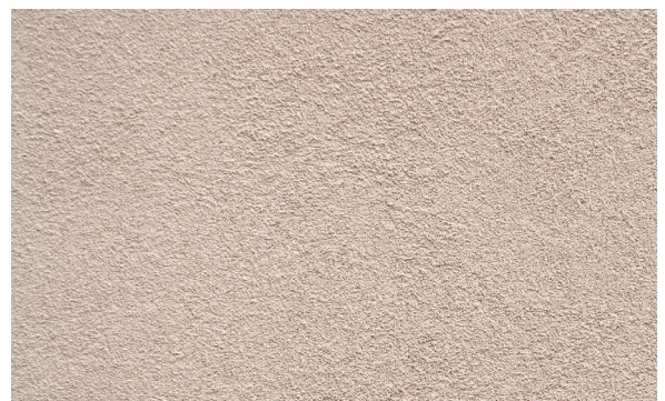
10. Final finishing of the PX-20 Isolxtrem RTX F.
