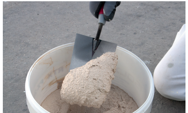
2. Remove the PX-20 Isolxtrem RTX F with the help of a pallet.
